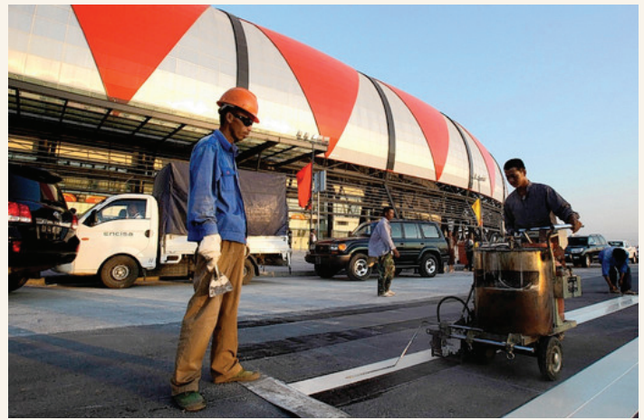
Chinese workers paint lines onto a crosswalk outside the November 11 stadium
